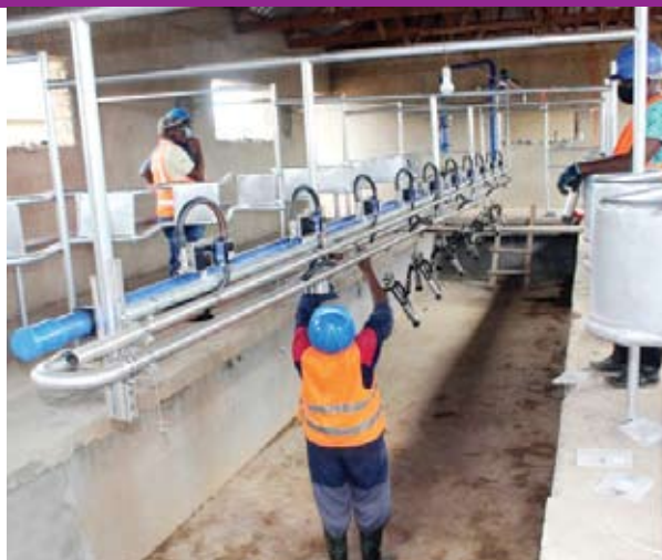
The milking parlour at Kasolwe stock farm equipped with a 10-line swing-over pipeline milking system
